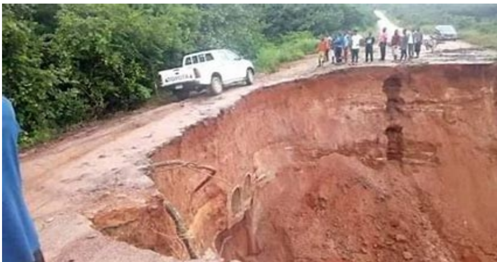
A gully erosion site in Isuikwuato LGA
